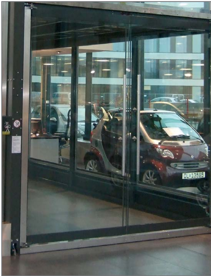
glass swing door in the first floor
