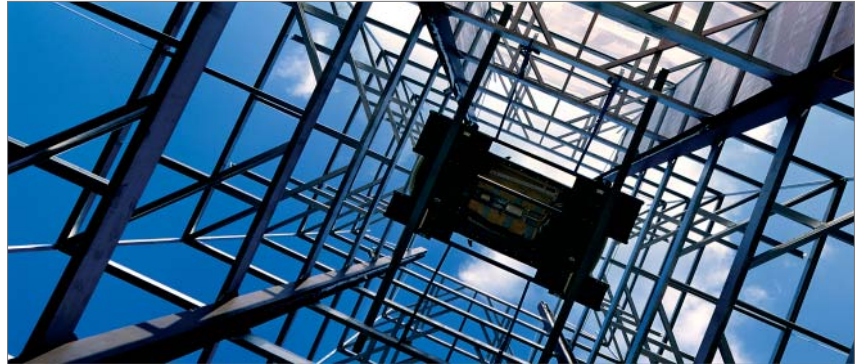
shuttle lift for transportation of the vehicles
